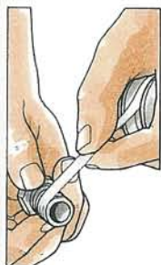
3 Taping the threads Make the threaded joints watertight by wrapping four or five turns of PTFE tape round the plugs and adaptors before you screw them into the new radiator. Use a hacksaw blade to roughen the threads, in order to encourage the tape to grip.
