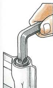
1 Removing the plugs Use a radiator spanner to unscrew the two blanking plugs at the top of the radiator.
