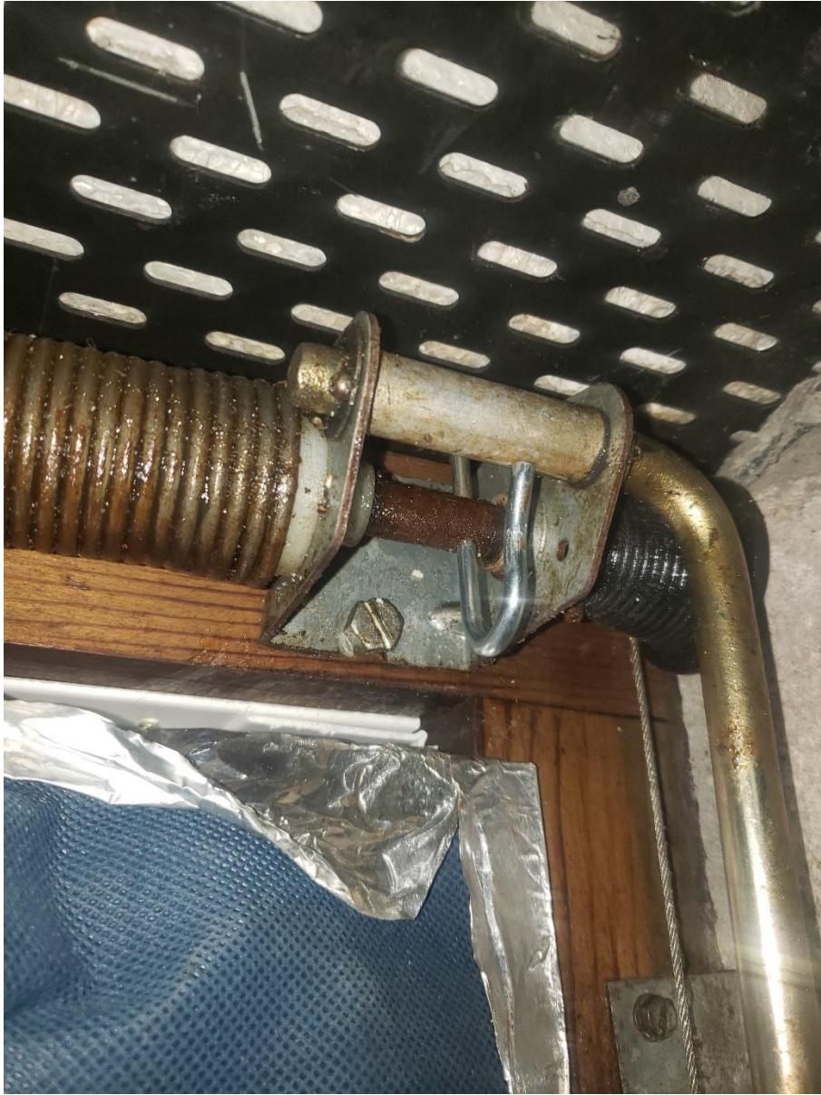
Figure 1-existing positionn of the crook pin (abutts the tube)
