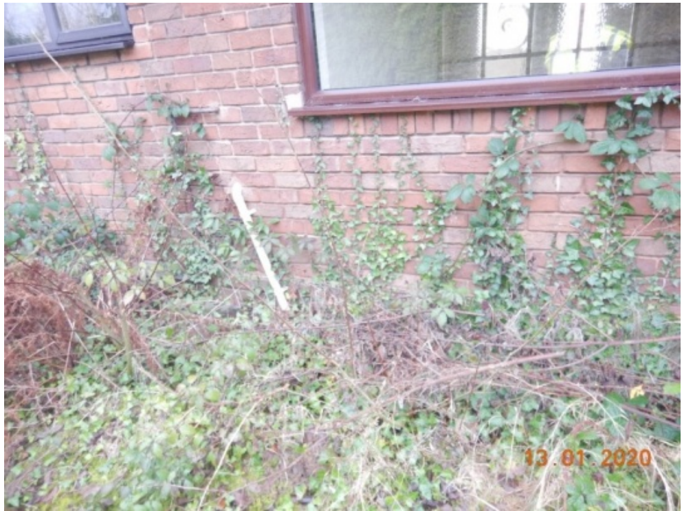
ivy to front and side walls
