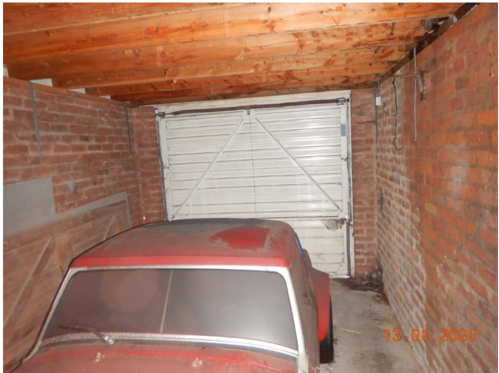
View inside garage
