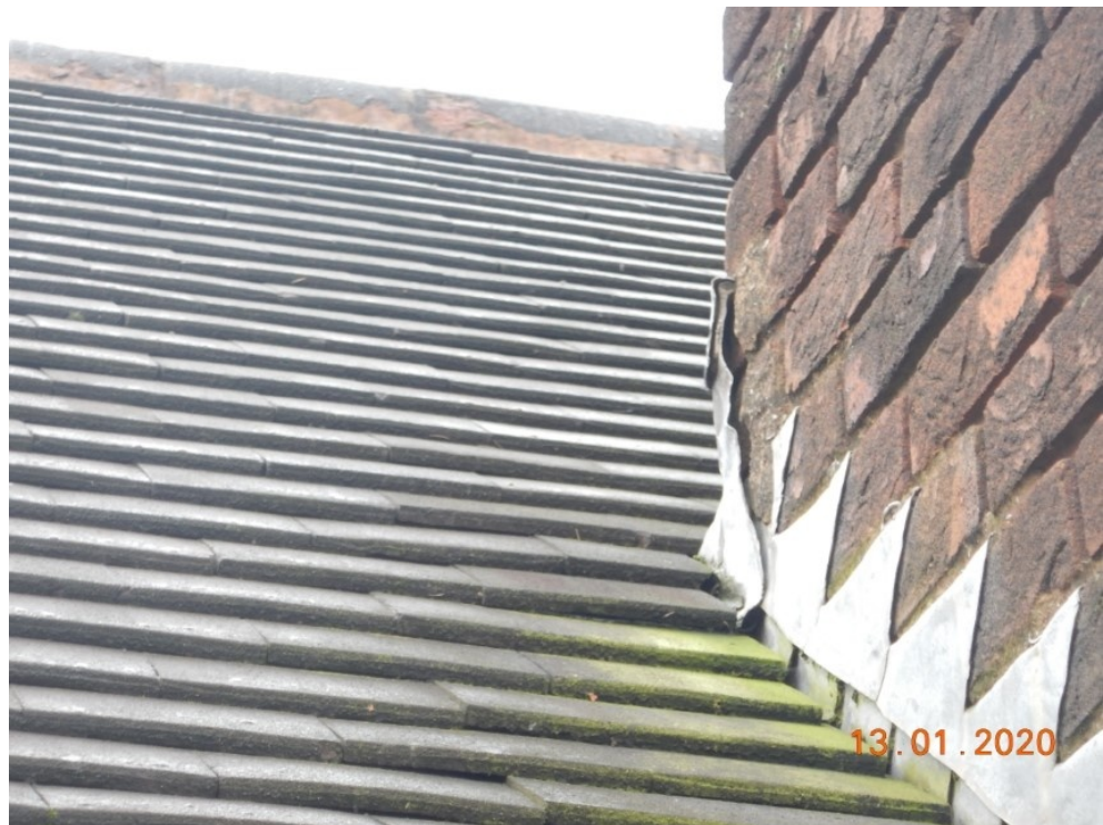
flashings lifting
