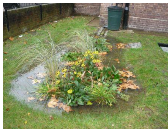
Unlined rain garden close to building foundations (deliberately filled for research)
