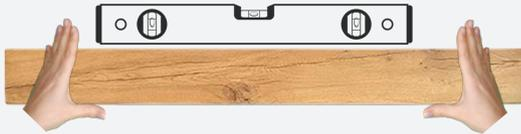
Push the beam all the way back on to the wall and gently level it using a spirit level, moving it gently into position. Keep the beam secure until it holds itself. (Usually around 5-7 minutes)
