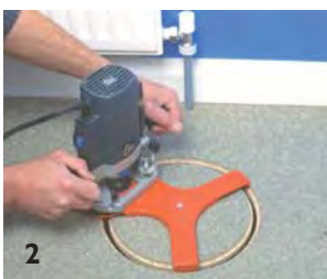
Routing the flooring sheet using the Routabout Rotating Template.
