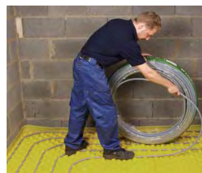
Laying Hep 2 O ® pipe
