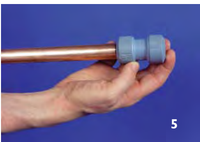
Push pipe firmly into fitting
