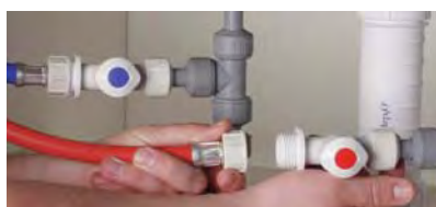
Connecting appliance valves
