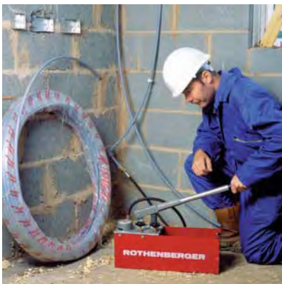
Setting up the pressure test
