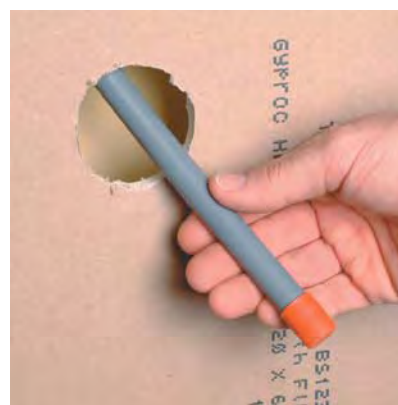
Fed pipe with end cap protection
