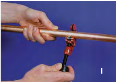
Cut copper pipe using a wheel cutter
