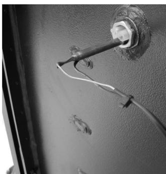
**Water temperature probe:** if the water temperature approaches the blocking temperature (85 °C), the probe requires to interrupt the supply of pellets.
