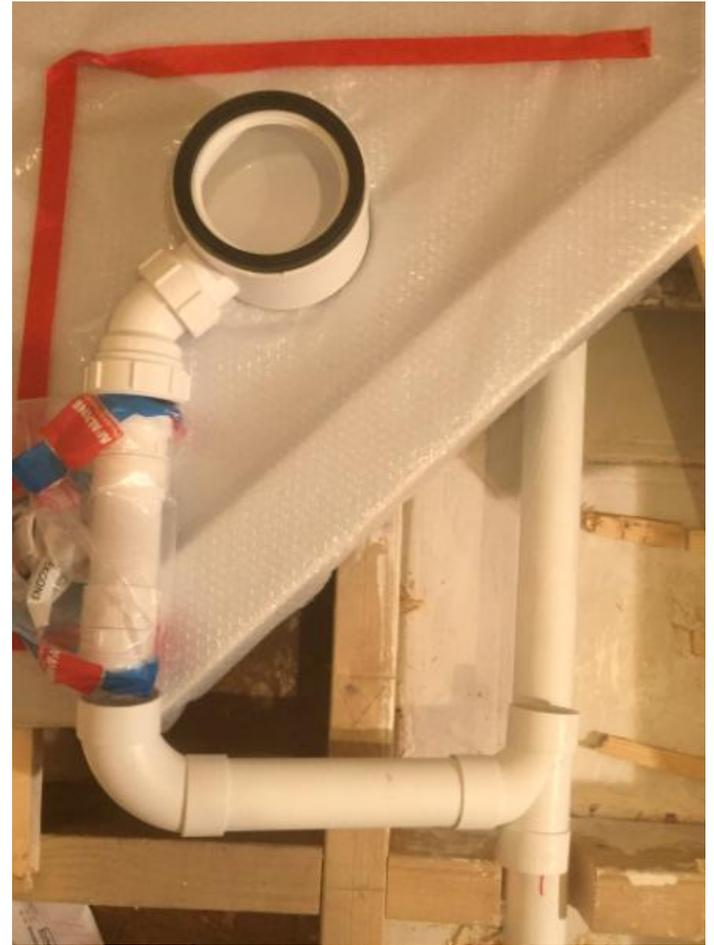
C. A longer route with flexing near the trap and rigid pipe with a sweep bend
