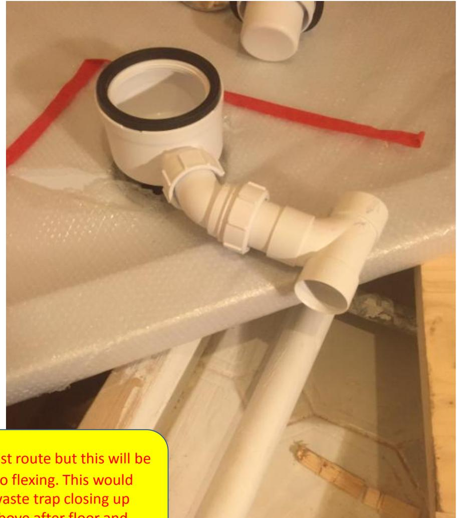
**A.** Shortest route but this will be rigid, no flexing. This would need waste trap closing up from above after floor and shower tray are laid.
